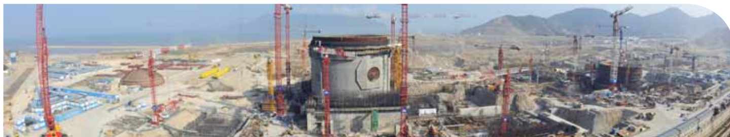
General View of Taishan Units 1 & 2 construction site - May 2011
