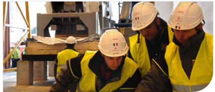
Teams preparing the RCP installation
