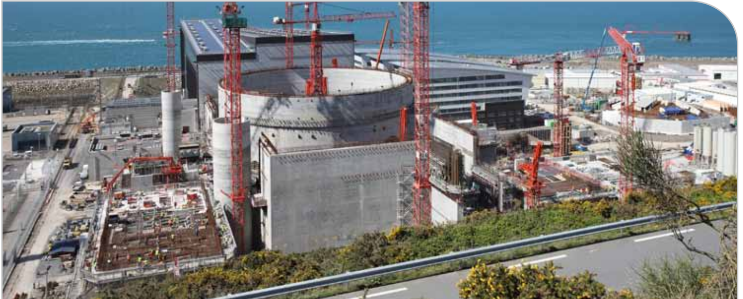
Flammanville 3 construction site - April 2011 - ©EDF
