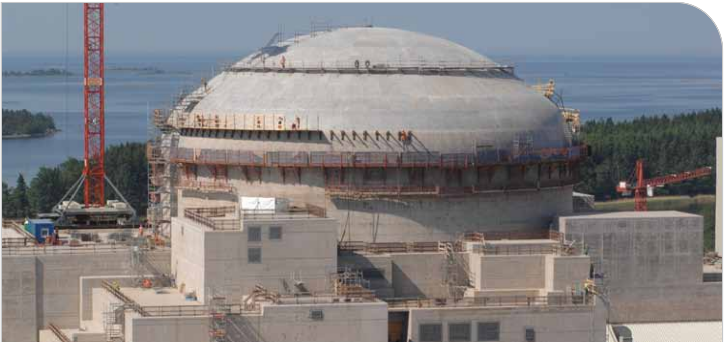
General view of Olkiluoto 3 construction site, Finland - May 2011
