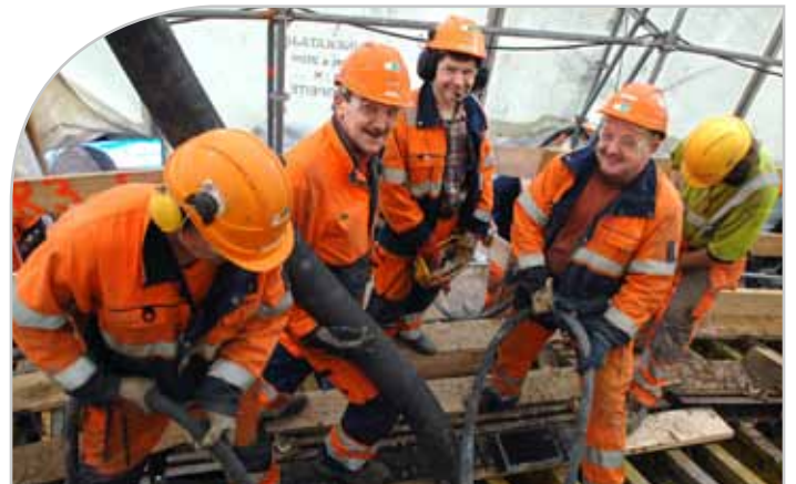
APC shell concreting operations
