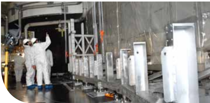
Launch of the implementation of the first Bertin filters in the IRWST
